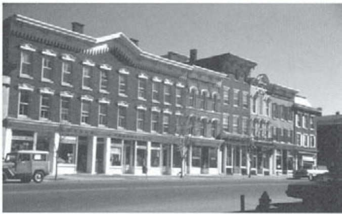
Fig. 2. Cazenovia, New York. Preservationists encouraged restoration of fine 19th century commercial buildings through an early façade improvement program.
